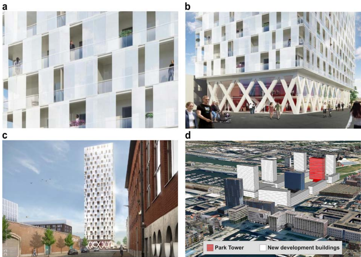
Figure 1. (a) Building facade with second-skin staggered facade concept. (b) Bottom of Park Tower with the second-skin concept, view from south-east. (c) Full view from south. (d) View of Park Tower (red), other new buildings under development (white) and already existing urban surroundings at the time of writing this paper.
